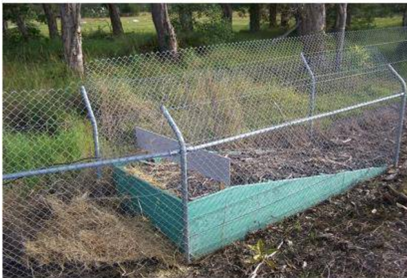
Figure 9.1.23 Retrofit fauna escape ramp.
