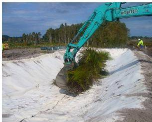
Figure 9.1.25 b) Slabbing method used to transfer wetland vegetation.
