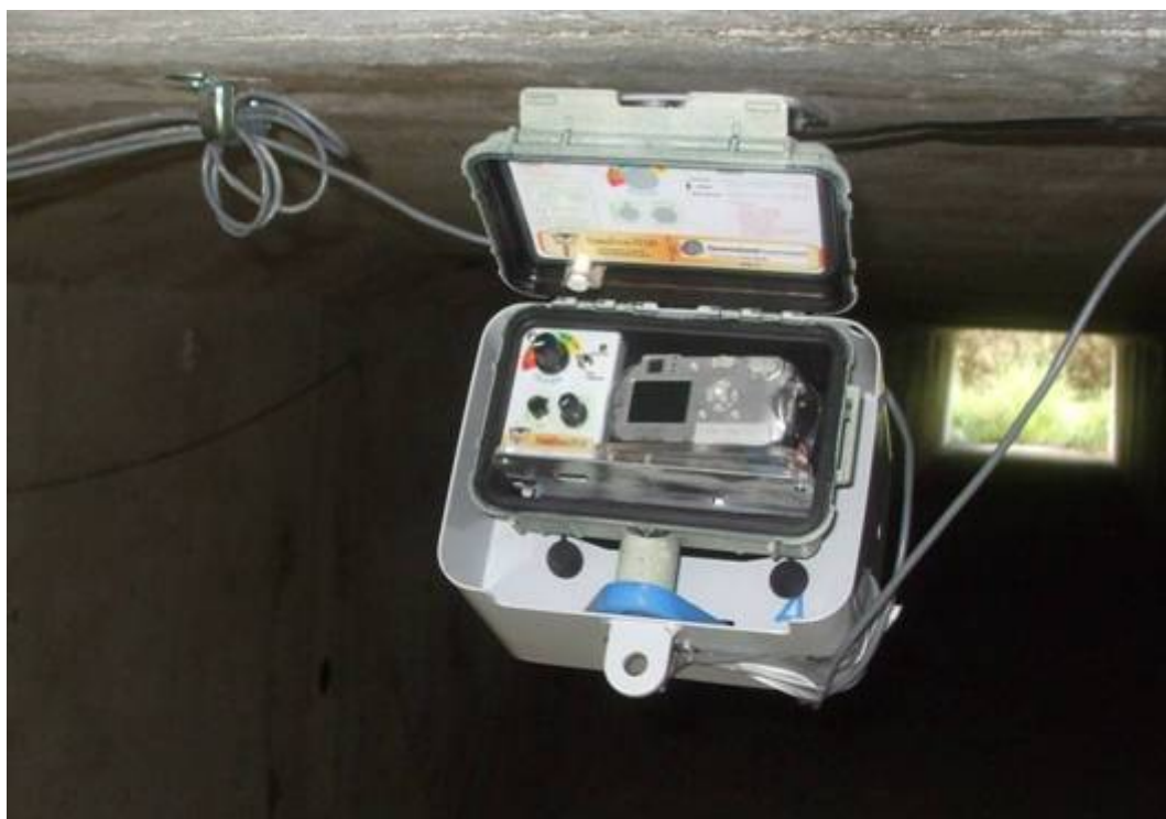
Figure 9.1.5 Infra-red still camera utilised in Boyd Street culvert
