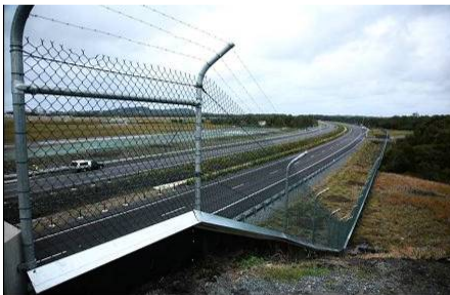
Figure 9.1.19 a) Frog fence attached to floppy top fencing.
