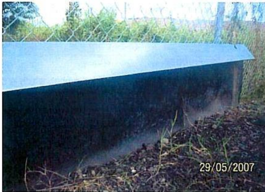
Figure 9.1.19 b) Permanent frog fence design to be attached to the existing airport security fence (PacificLink Alliance 2007).
