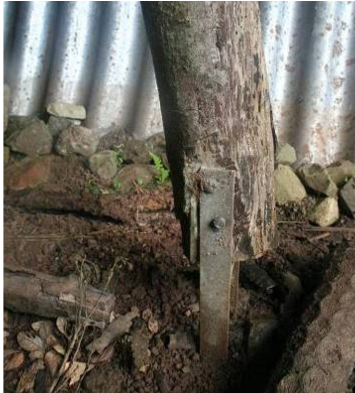
Figure 9.3.3. Footings for underpass furniture (Scott 2008).
