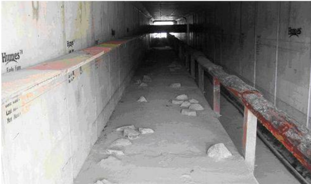
Figure 9.2.6 An underpass at Compton Road. Note the raised cement level with rock ‘furniture’, wooden shelf and log railing (Bond and Jones 2006).
