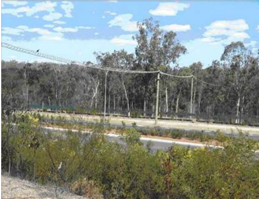
Figure 9.2.10 Canopy bridge used by arboreal species to the road (Scott 2007).
