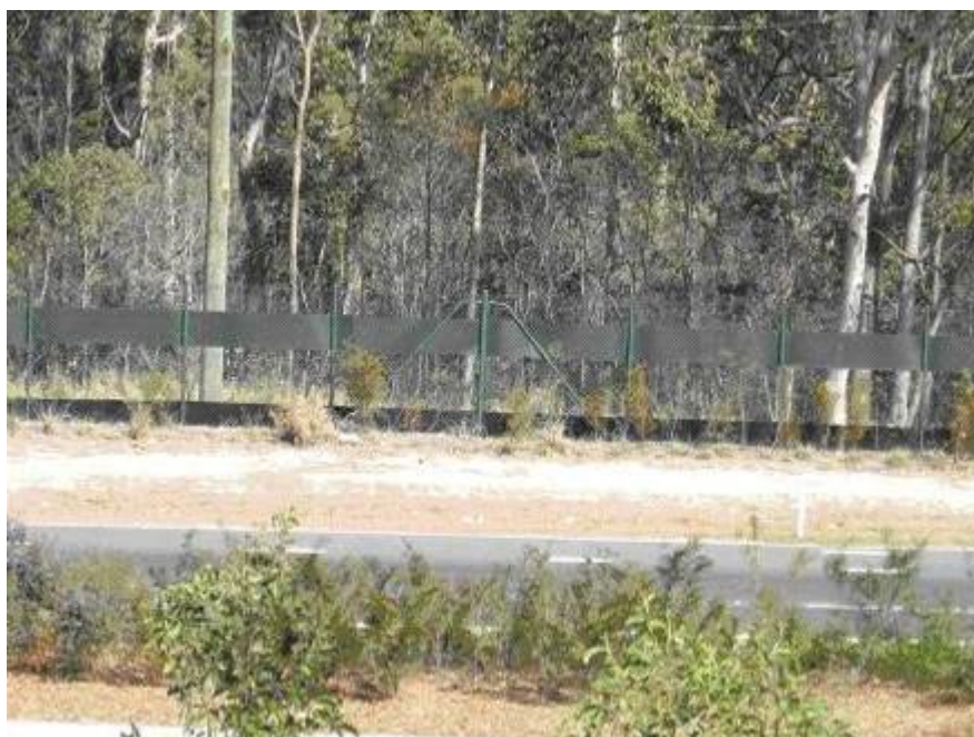
Figure 9.2.5 Fauna exclusion fencing at Compton Road (Robinson-Wolrath 2008).
