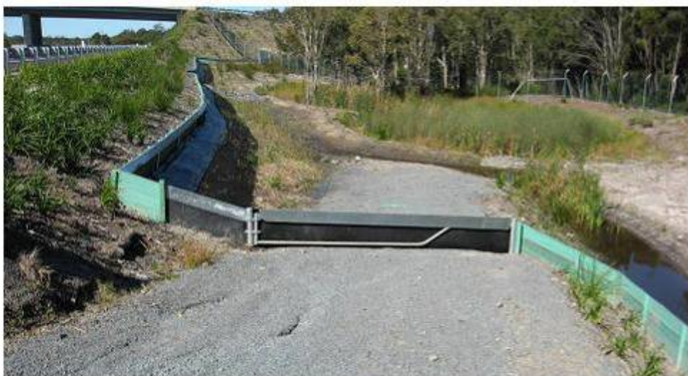
Figure 9.1.16 Specially designed frog gate across access track. Note the geofabric at the base of the frog fence.
