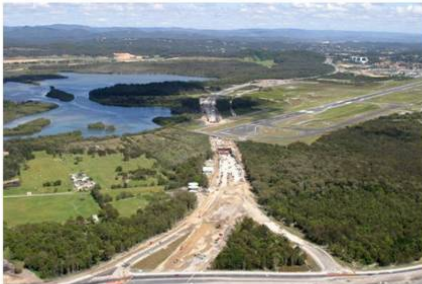
Figure 9.1.1 Tugun Bypass project under construction.
