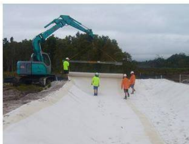
Figure 9.1.25 Frog pond construction process.
