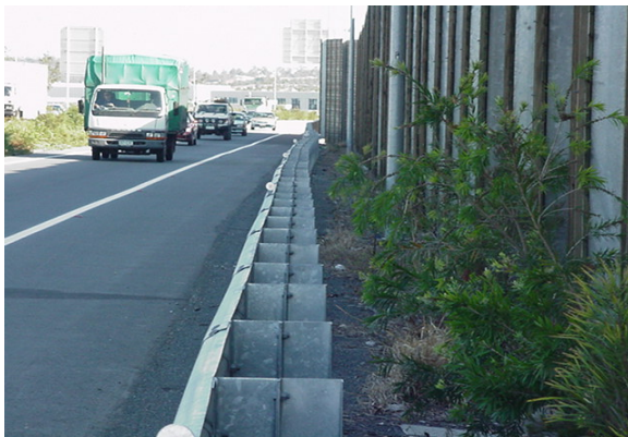
Figure 2 (b) - Use of standard noise fence with narrow setback creates undesirable visual effect
