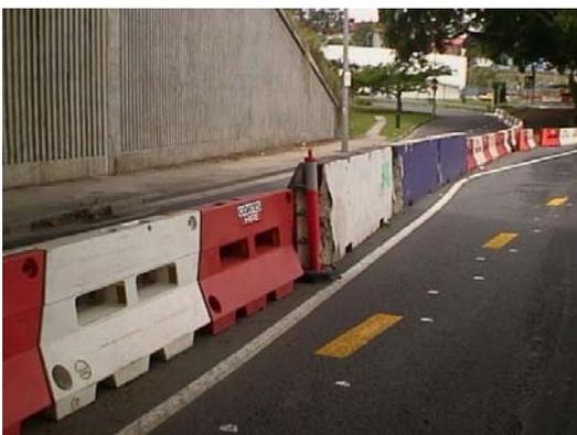
**Figure 8.127** This is not adequate as a barrier system; neither the plastic blocks nor their arrangement comply with the requirements for re-directive barriers or end treatments under AS3845
