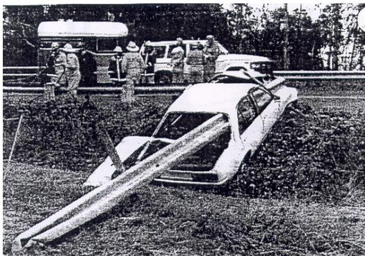
**Figure 8.82** This is the reason for moving to the MELT system as given in the current Main Roads Standard Drawings for guardrail
