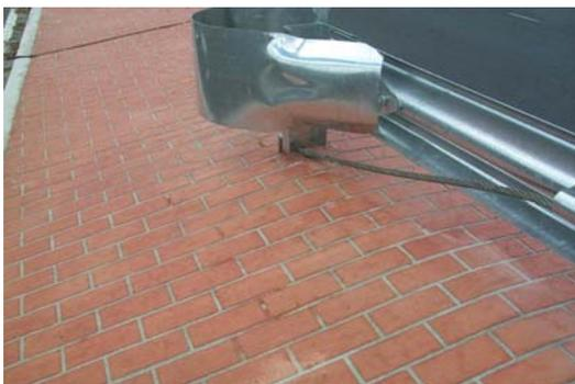
**Figure 8.94** Slip base mechanism, probably installed correctly, which has been rendered inoperative by the addition of decorative concrete overlay
