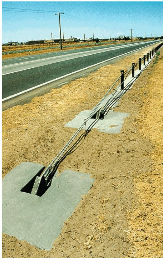
**Figure 8.77** Wire rope end treatment showing below ground anchorage
