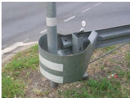
**Figure 8.96** The traffic signals post will prevent this end treatment from operating in the desired manner
