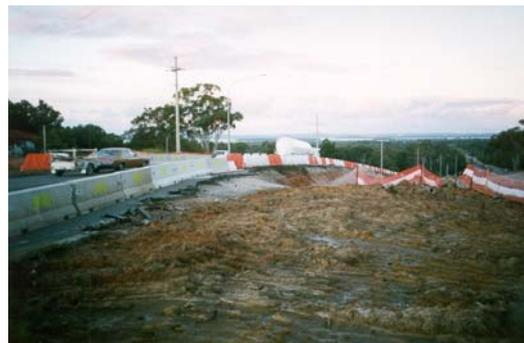
**Figure 8.129** The temporary plastic blocks will not redirect errant vehicles
