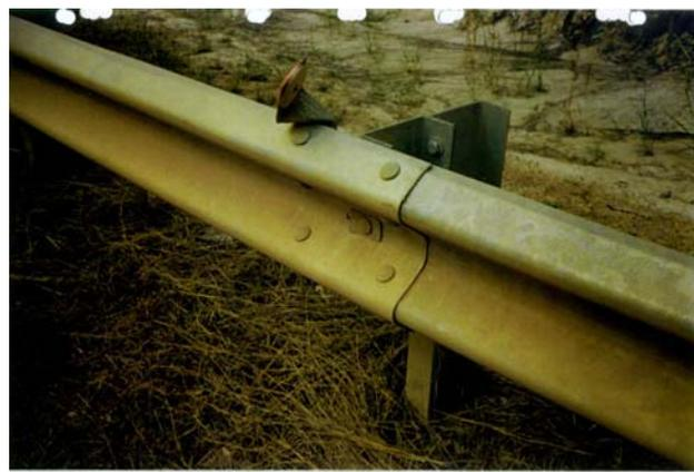
**Figure 8.93** Poor installation practice
