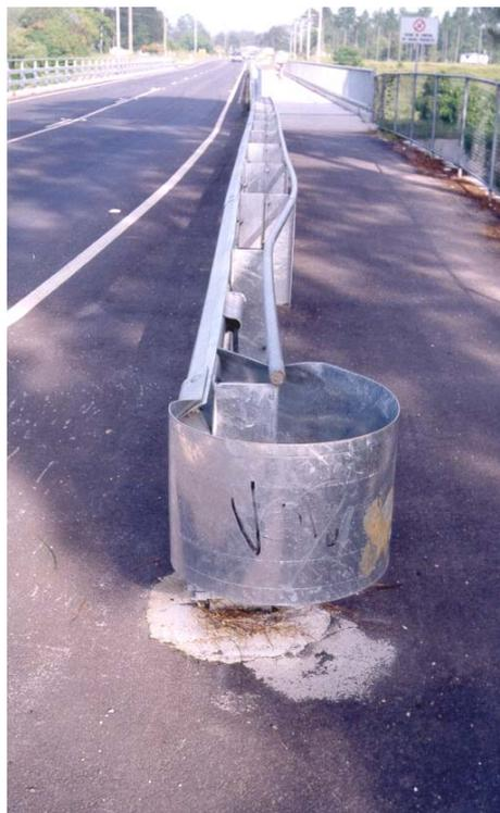
**Figure 8.80** Spearing hazard created by welding a bar (A) to the back of an end treatment in an attempt to make the posts more friendly to pedestrians and cyclists
