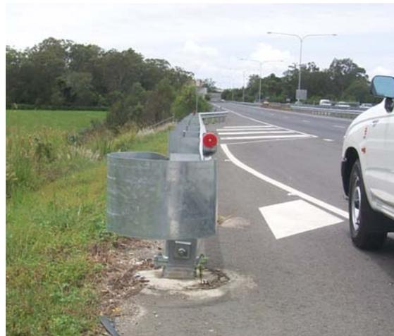
**Figure 8.105** Dead straight end rails, no offset, no flare, no curve; a spearing hazard regardless of the mass of the impacting vehicle.
