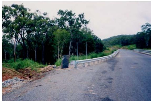
**Figure 8.101** Incorrect installation – no hazard free zone
