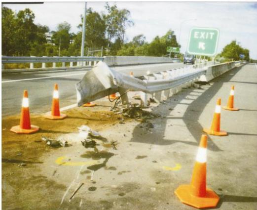
**Figure 8.107** Showing a back-to-back w-beam end treatment after crash
