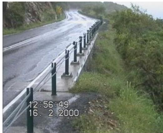
**Figure 8.117 An innovative approach to installing wire rope barriers at a difficult site whilst preserving the scenic character**
