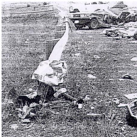
**Figure 8.84** The failure of the end treatment to operate when hit in the fatality shown in Figure 8.83 can be seen here
