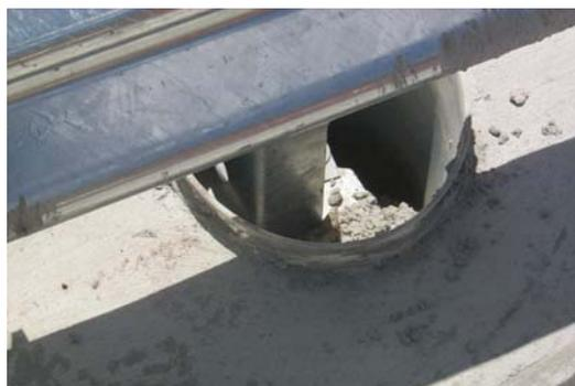
**Figure 8.98** Close-up of slip base arrangement from Figure 8.97
