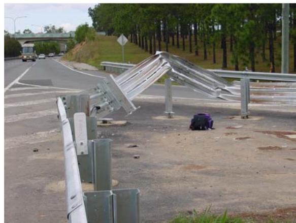
**Figure 8.88 Thrie-beam bullnose – gore area, after initial impact**
