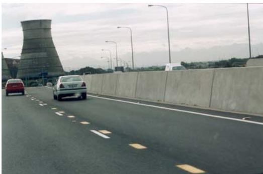
**Figure 8.126** Single slope rigid barrier system used as a median barrier
