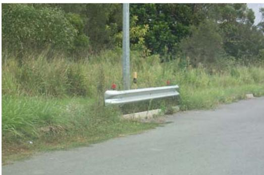
**Figure 8.123** This short section does not have anchored ends and is too short
