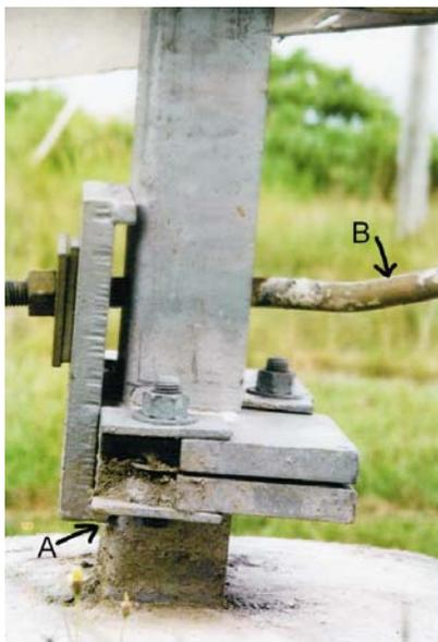
**Figure 8.78** Illustrating general but sub-optimal arrangement for w-beam slip base assembly
