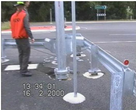
**Figure 8.99** This barrier has been incorrectly installed on the side leg of a T-junction
