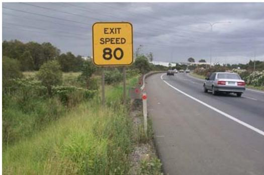
**Figure 8.103** This installation did not comply when built – incorrect offset
