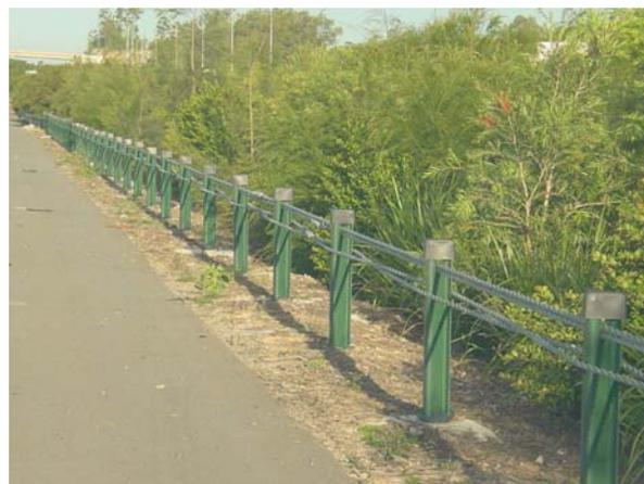
**Figure 8.118 Wire rope barrier**
