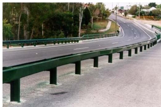
**Figure 8.125** Light steel sheeting covering the pedestrian/cycle side of w-beam guardrail installation
