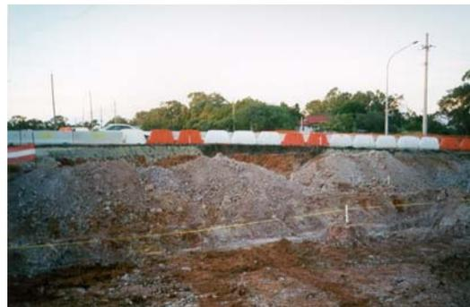
**Figure 8.130** This drop (of about 12m) is the reason the temporary plastic blocks were installed (Figure 8.129)
