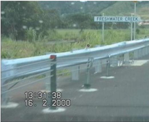
**Figure 8.131** Transition between w-beam bridge approach and wire rope barrier
