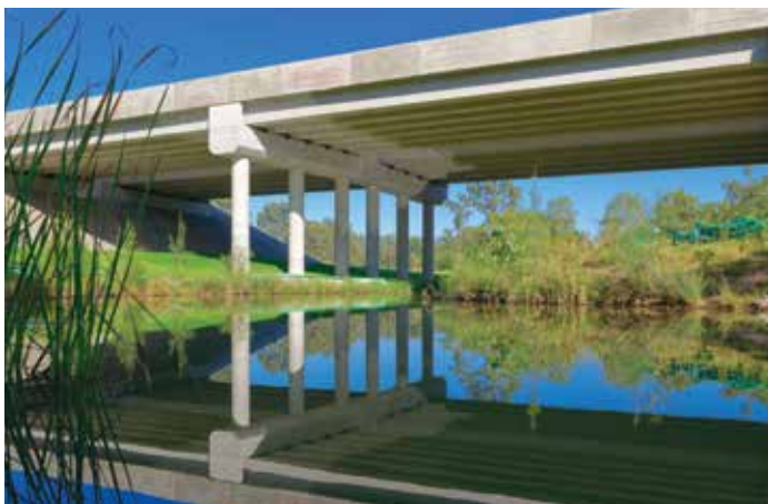
Traveston Creek Bridge on Section C: Traveston to Woondum showing revegetated creek banks
