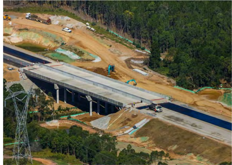
Progress of Cobbs Gully bridge and pavement works
