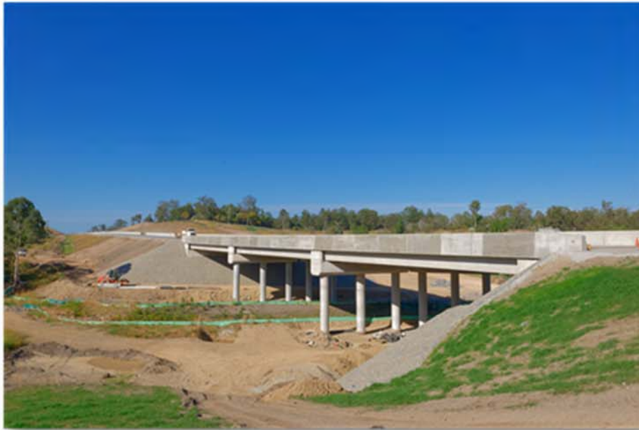
New Cobbs Gully Bridge and diversion
