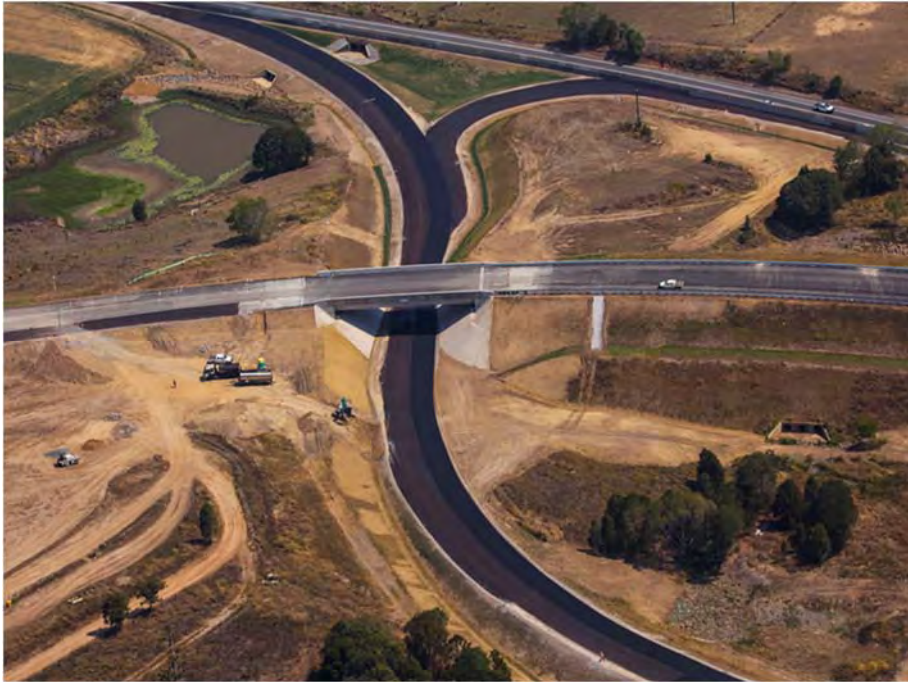
Progress of northern connections at Woondum (October 2017)
