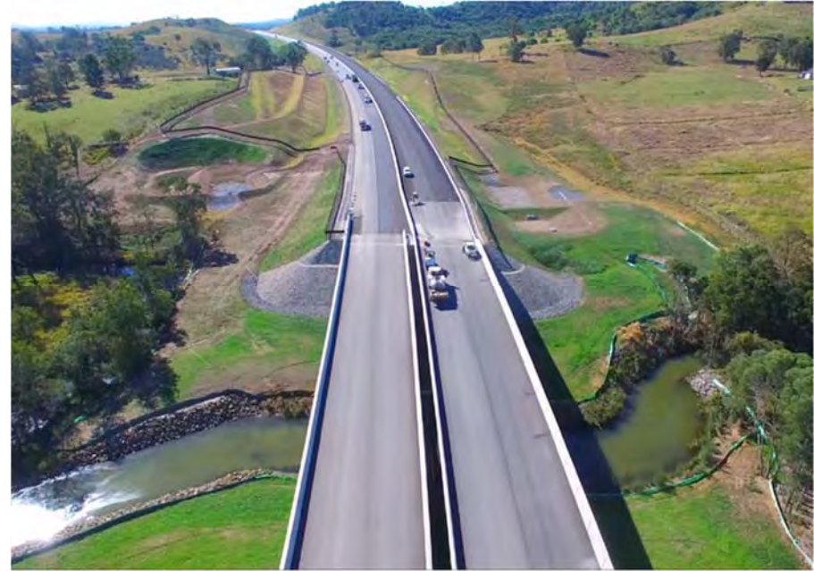
Completed Traveston Creek realignment and bridges – looking north (August 2017)
