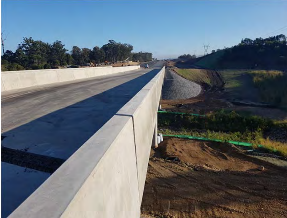
Looking north across the Jackass Creek Bridge (June 2017)
