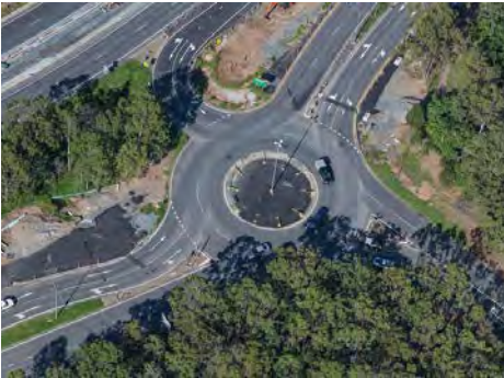
Bracken Ridge Road and Barfoot Street intersection works
