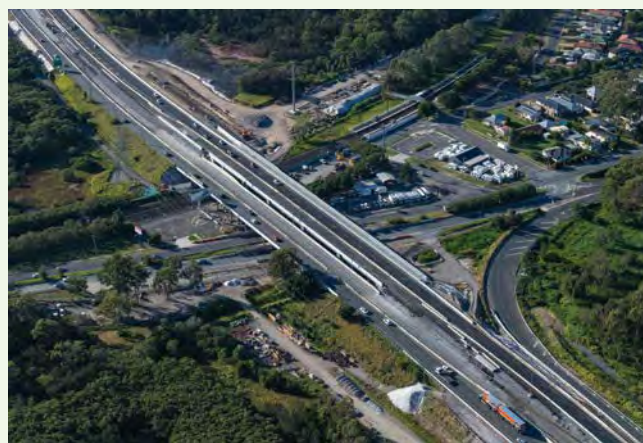
The upgraded Sandgate Road bridge
