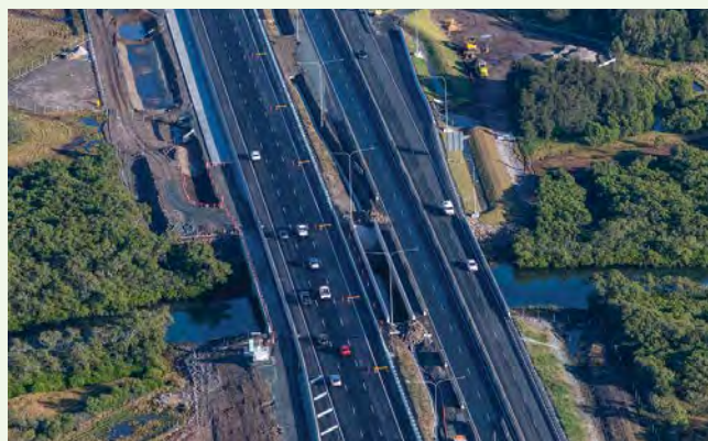
The upgraded Nundah Creek bridges
