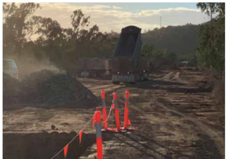
Earthworks on the Nora Road extension
