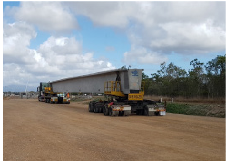
A truck waiting to deliver a girder to site.
