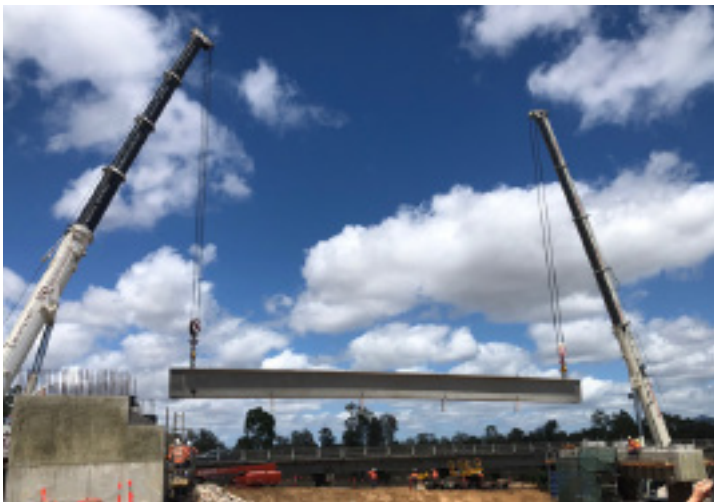
Two specialised cranes are used to install the 84 tonne girders
