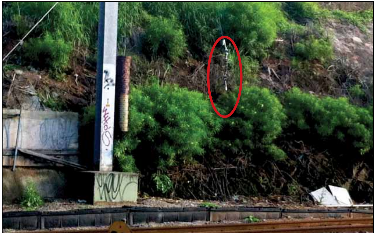
Figure 6 - Dislodged OHLE.
