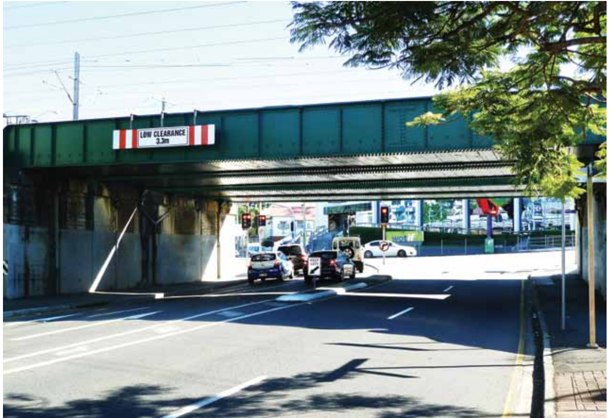
Figure B7 – Park Road Bridge from Park Road, Milton.
